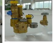
Multivalve REGO or OMECA combines double back check filler valve, vapour equalizing valve with excess flow, pressure relief valve, service shut-off valve, Junior level gauge and pressure gauge. Additionally installed is liquid service valve.
